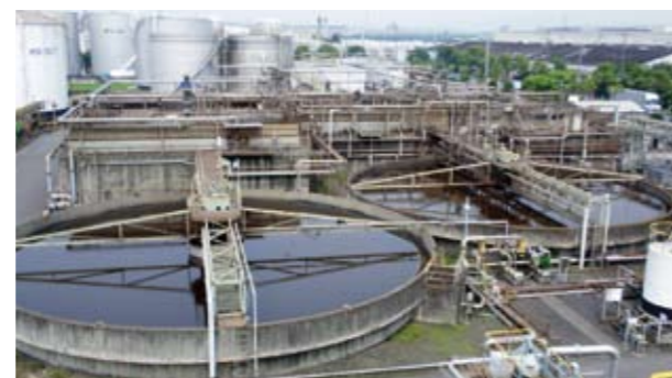
Mizushima Plant activated sludge treatment equipment
