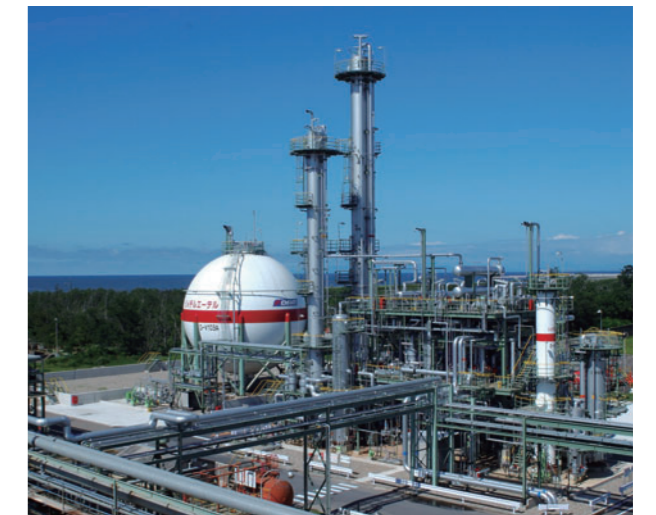
Fuel DME Promotion Plant inside MGC's Niigata Plant
